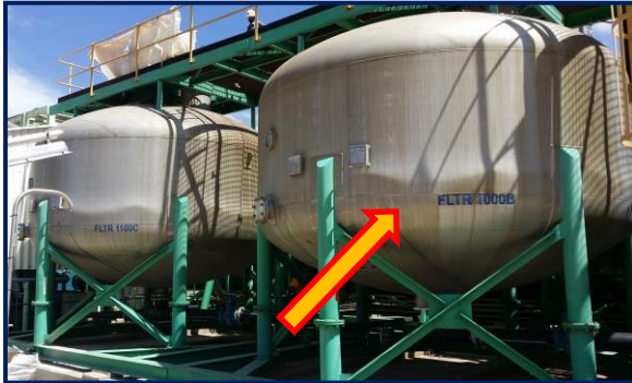
Gypsum accumulation bending steel structure of activated carbon electrolyte filter
